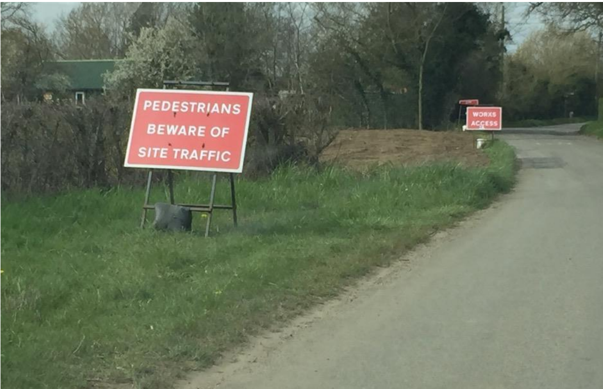
Photo 8 – Site entrance from Grove Road (3 of 4) near Fareacre
